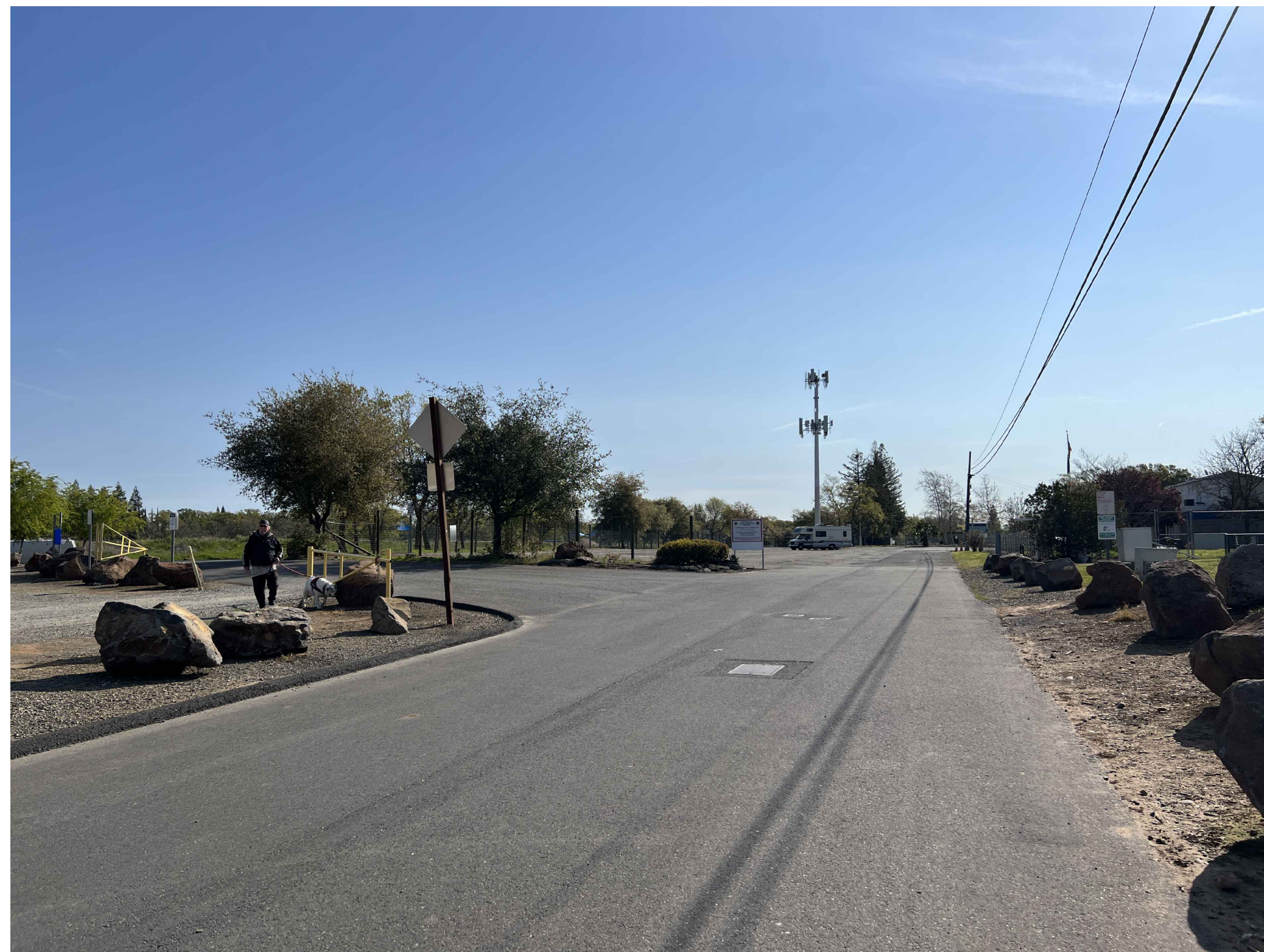
5 VIEW EAST TO VEHICULAR ACCESS, VFW ENTRY AND CONNECTION TO MAYA STREET
