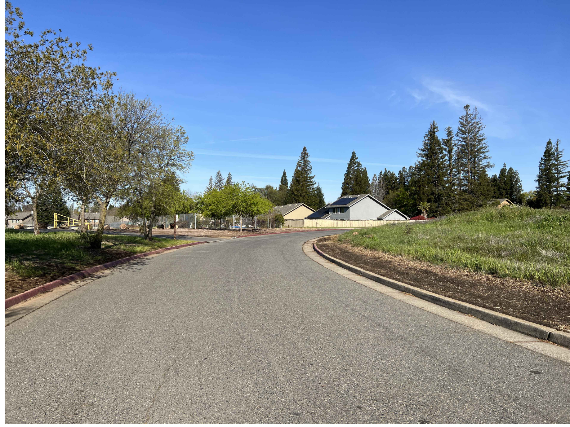
1 MAYA STREET FRONTAGE LOOKING WEST
